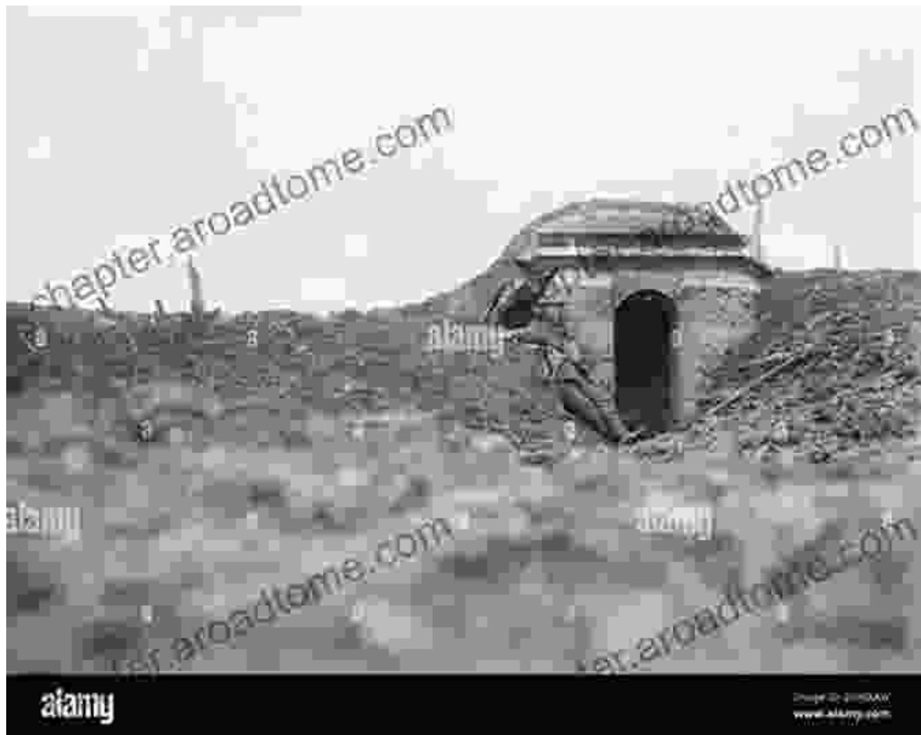
The fortifications of the Hindenburg Line were designed to maximize German defensive capabilities. Bunkers and pillboxes, made of reinforced concrete, provided protection for troops and machine gun nests, creating formidable strongholds along the front.
